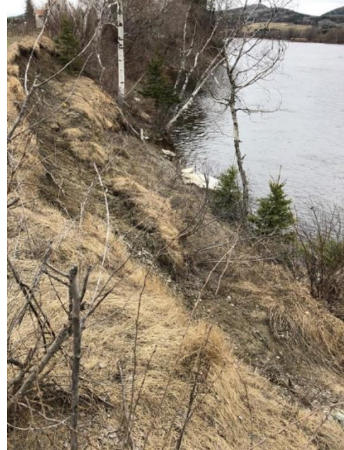
Figure 6: Existing slope condition on section East of Frenchville
