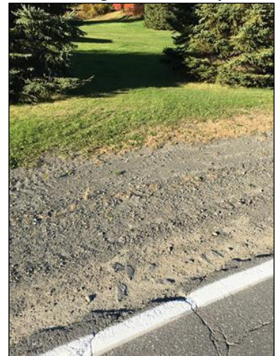
Figure 2: (left) Road surface cracking and breaking apart near edge, creating instability for vehicles, bicycles, and pedestrians using shoulder. (Right) Gravel shoulder compromised by erosion, wash boarding, and pavement cracking.
