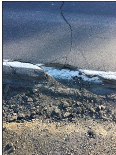
Figure 2: (left) Road surface cracking and breaking apart near edge, creating instability for vehicles, bicycles, and pedestrians using shoulder. (Right) Gravel shoulder compromised by erosion, wash boarding, and pavement cracking.
